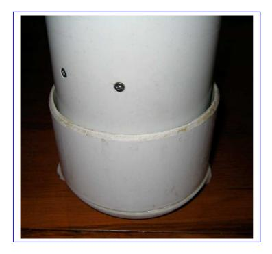
The photo to the left shows the PVC shield fitted, prior to the Pozidrive screws being bored and then self tapped into the zinc.
